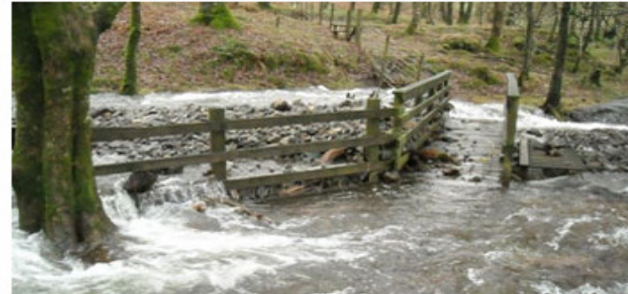
A flooded bridge near Coniston.
